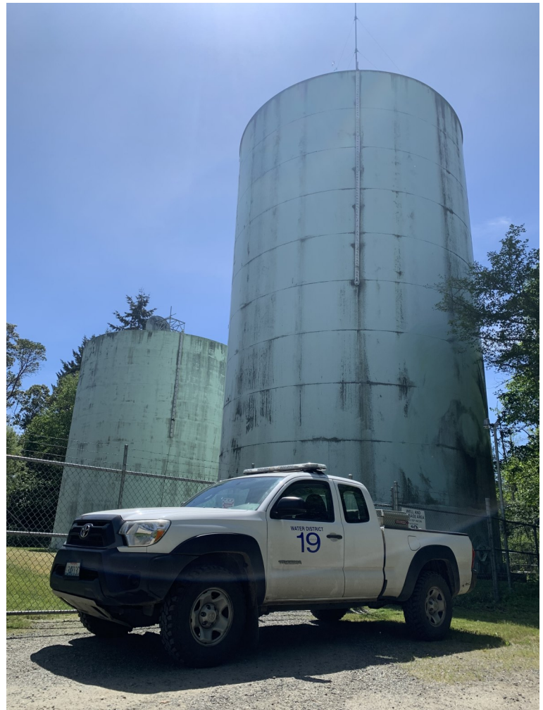
Million gallon & 625K tank at wellsite
